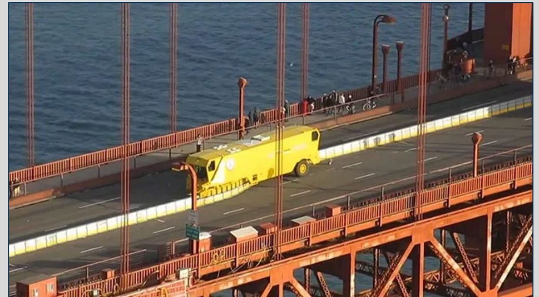
Golden Gate Bridge Moveable Barrier Project, 2012
