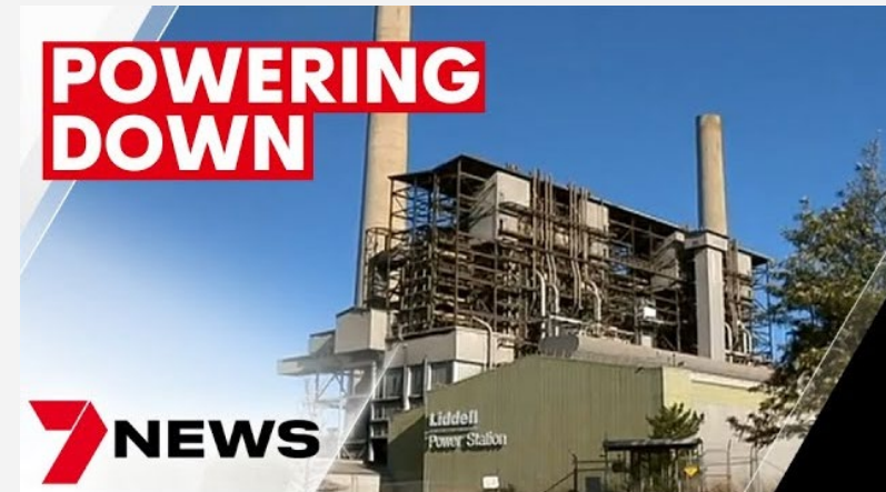
Liddell coal station (NSW) closed in May (~1600MW)
