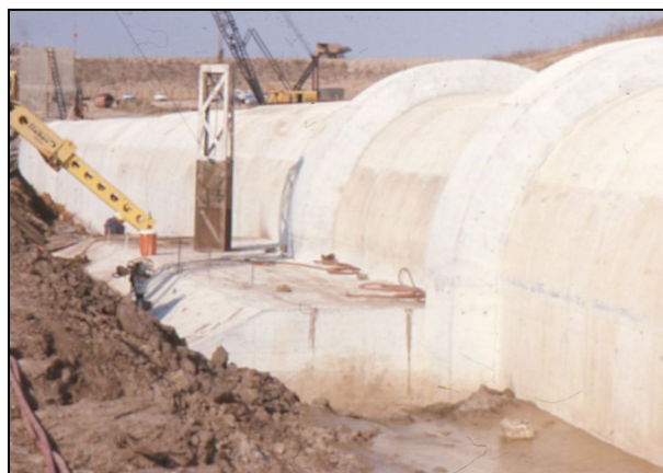
Portion of concrete plug along conduit (outlet works station 50+00 and dam station 71+50)
